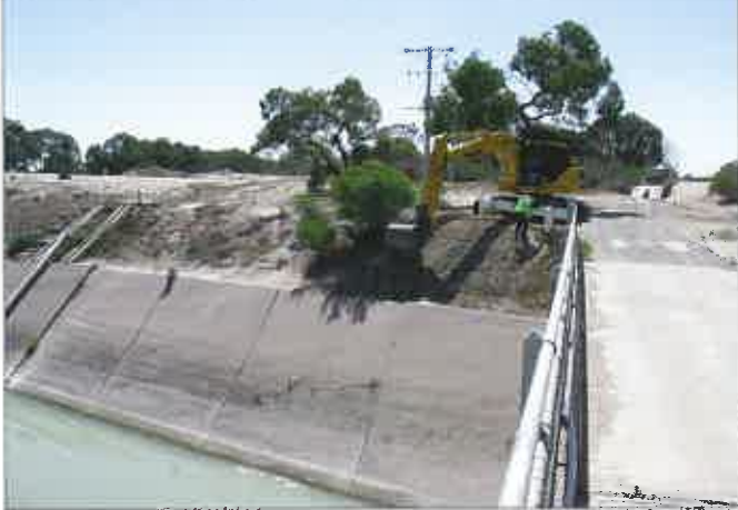
The PC160-7 in batter cleaning work.
