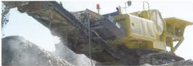
Army crusher working on Palm Island.
