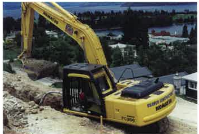
One of Beaver Contractor's fleet of Komatsu excavators and loaders.
