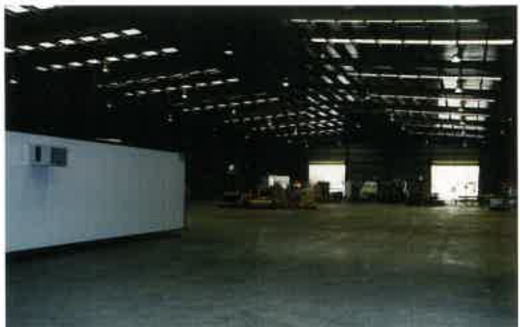
Space, space and more space. The inside of the new premises before the shelving and other trimming went in.
