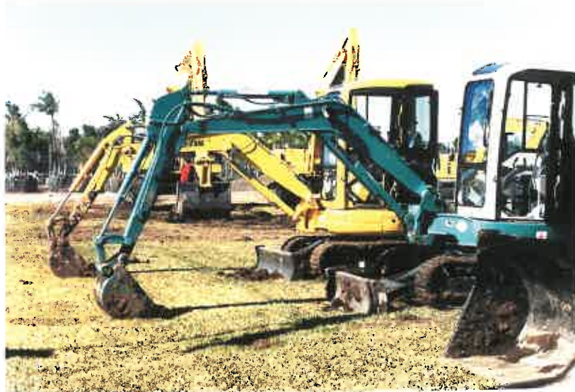
The mini excavator line up got a good workout as did the other machines on display at the Big Dig.
