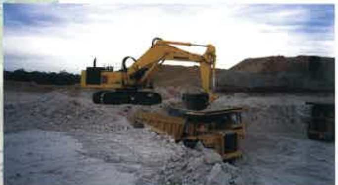
Right: Evanbank Plant Hire's two new machines working on-site at Wirralie Gold Mine.
