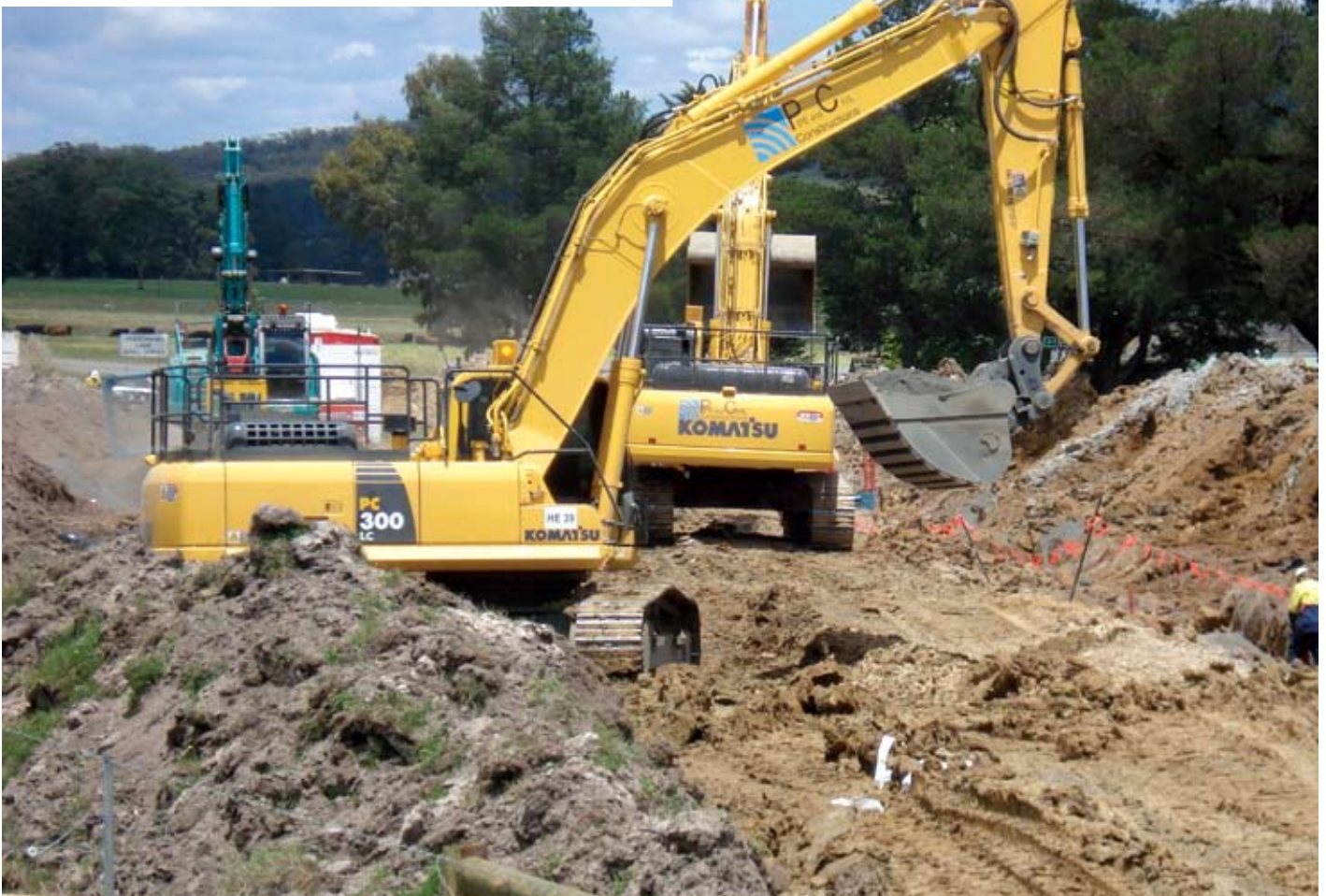
ABOVE/RIGHT. Victoria's Sugarloaf Pipeline Project.
