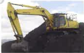
Singleton Earthmoving's PC450-6 carrying out clean up work at Bulga Coal.
