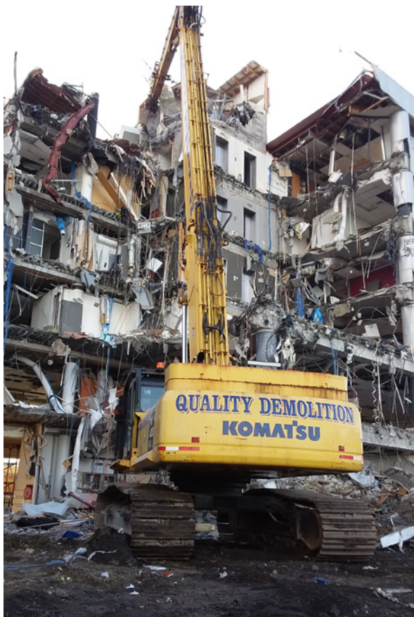
Pictured above: A PC400LC-8R working on removing the Wellington Electricity building's superstructure
