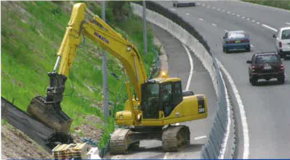
Austeire's PC200-7 working on the Lane Cove tunnel project
