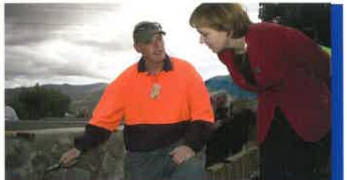
Stoneworks trainee Chris Slater shows Minister Lara Giddings the principles behind stone-faced concrete wall construction.
